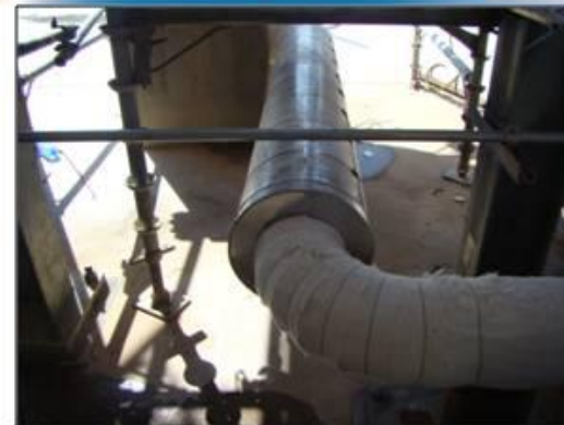
Perlite with cladding. 10mm Pyrogel XT (less cladding required)
